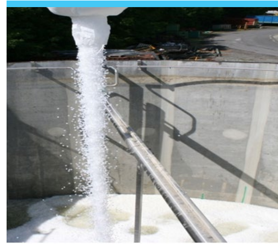
Biofilm being filled in wastewater tank.
